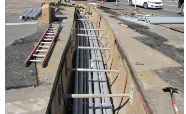
Lay conduit and encase in concrete
