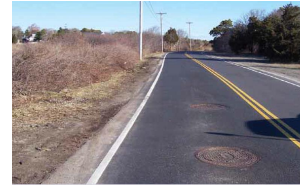
Final pavement with new asphalt
