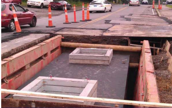
Installation of manholes
