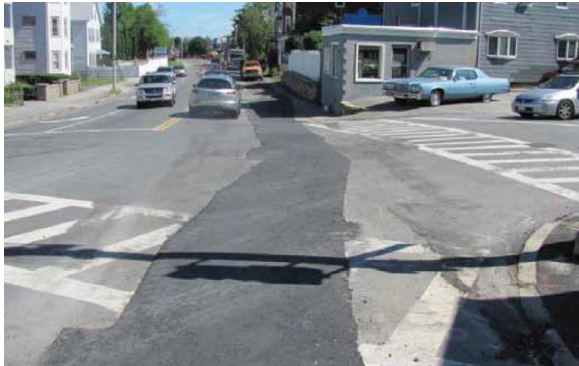
Backfill trench and install temporary pavement
