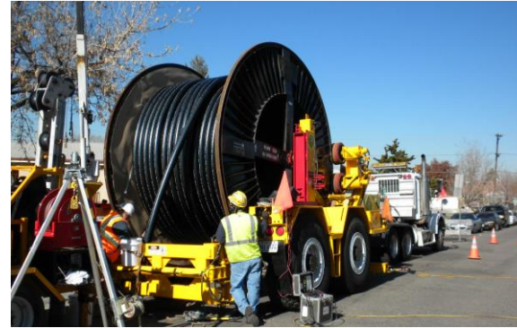
Pull and splice cable
